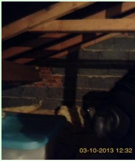
cavity block construction to gable ends
