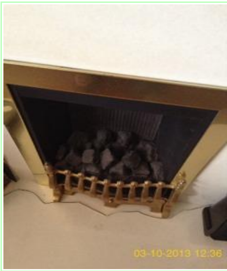
Flush fitting live fuel effect open front fire, sealed to fireplace
